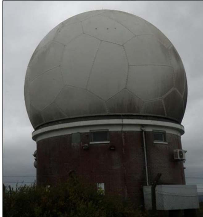
Figure 16. Woodcock Hill Radar Station
